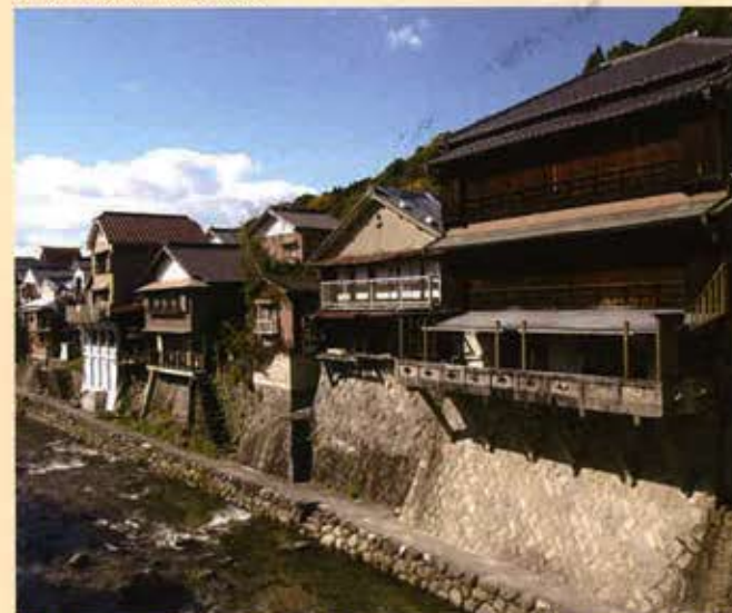
● The view from a top of the Mayumibashi Bldg, spanning the river.
